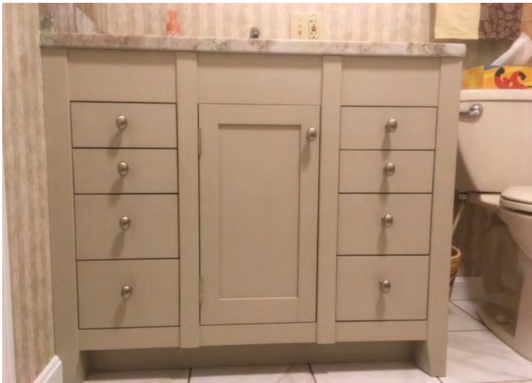
The 4 items shown are painted cabinet work. Below: Vanity cabinet with “flush drawer fronts.” Note the even spacing of the “flush fronts” that are most difficult to achieve (Ron Boes)
