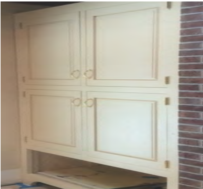
The 4 items shown are painted cabinet work. Below: Vanity cabinet with “flush drawer fronts.” Note the even spacing of the “flush fronts” that are most difficult to achieve (Ron Boes)
